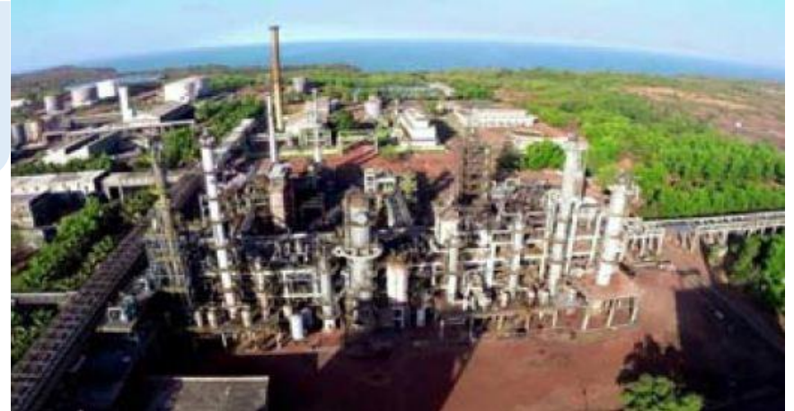
PVC resin Plant at Ratnagiri
