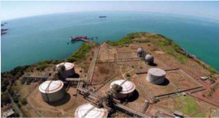
Storage tanks for raw material
