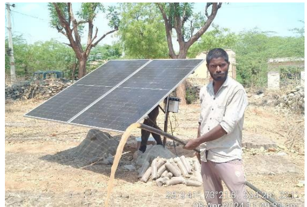
Installation of solar water pump sets that provide water for animals in Ranakpur Wildlife Sanctuary, Rajasthan.
